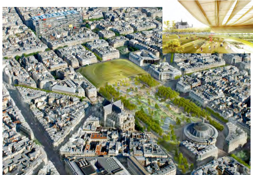
Figure Sixteen: Berger and Anziutti Canopy, under construction - 2012-2016.
