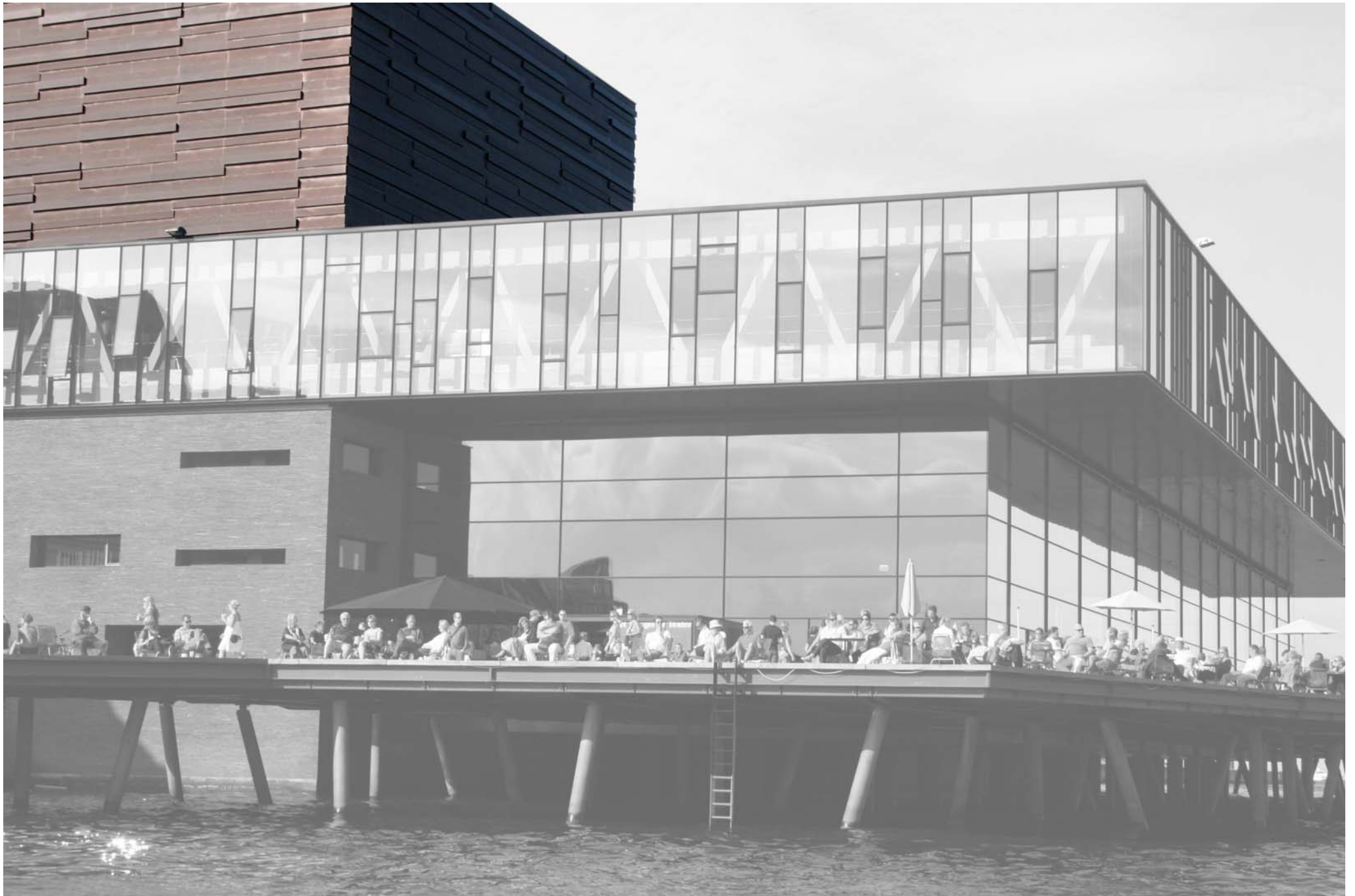
CONSTRUCTION & MATERIALS – Cooper clad fly tower
