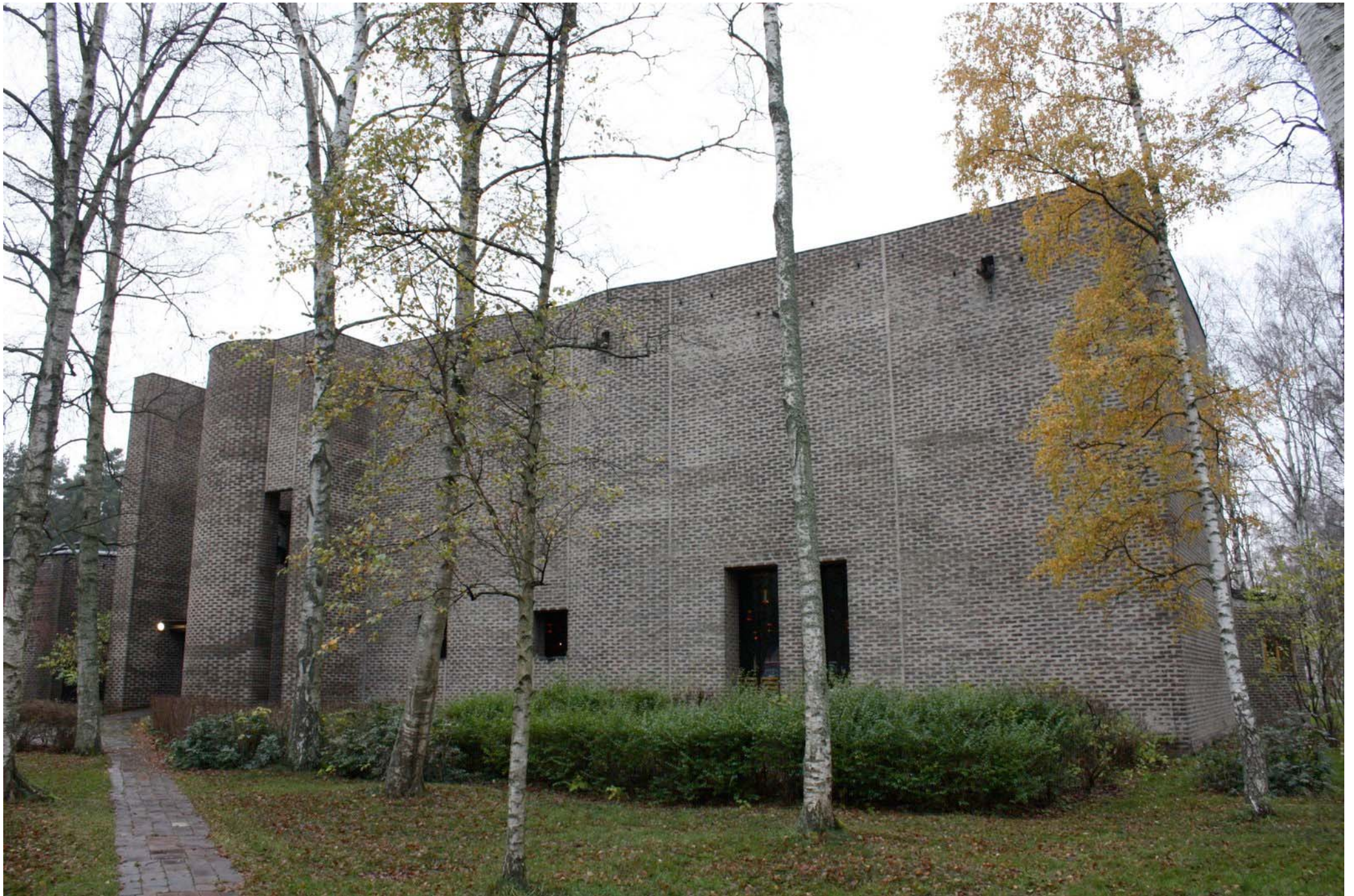
MATERIALS – Brick – Precedence – St Mark's Church (Sigurd Lewerentz)
