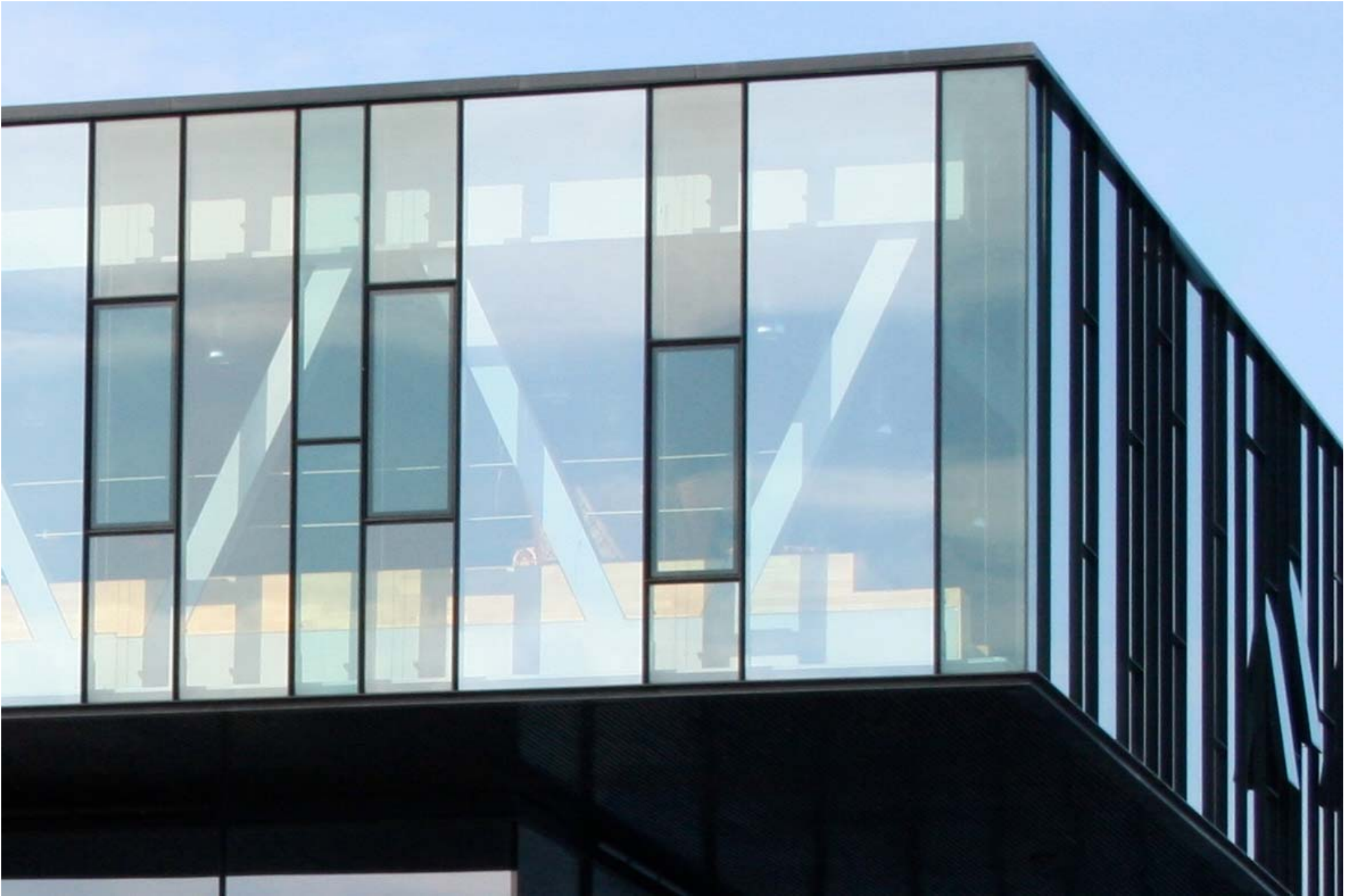
CONSTRUCTION & MATERIALS – Cantilevered all-glazed floor
