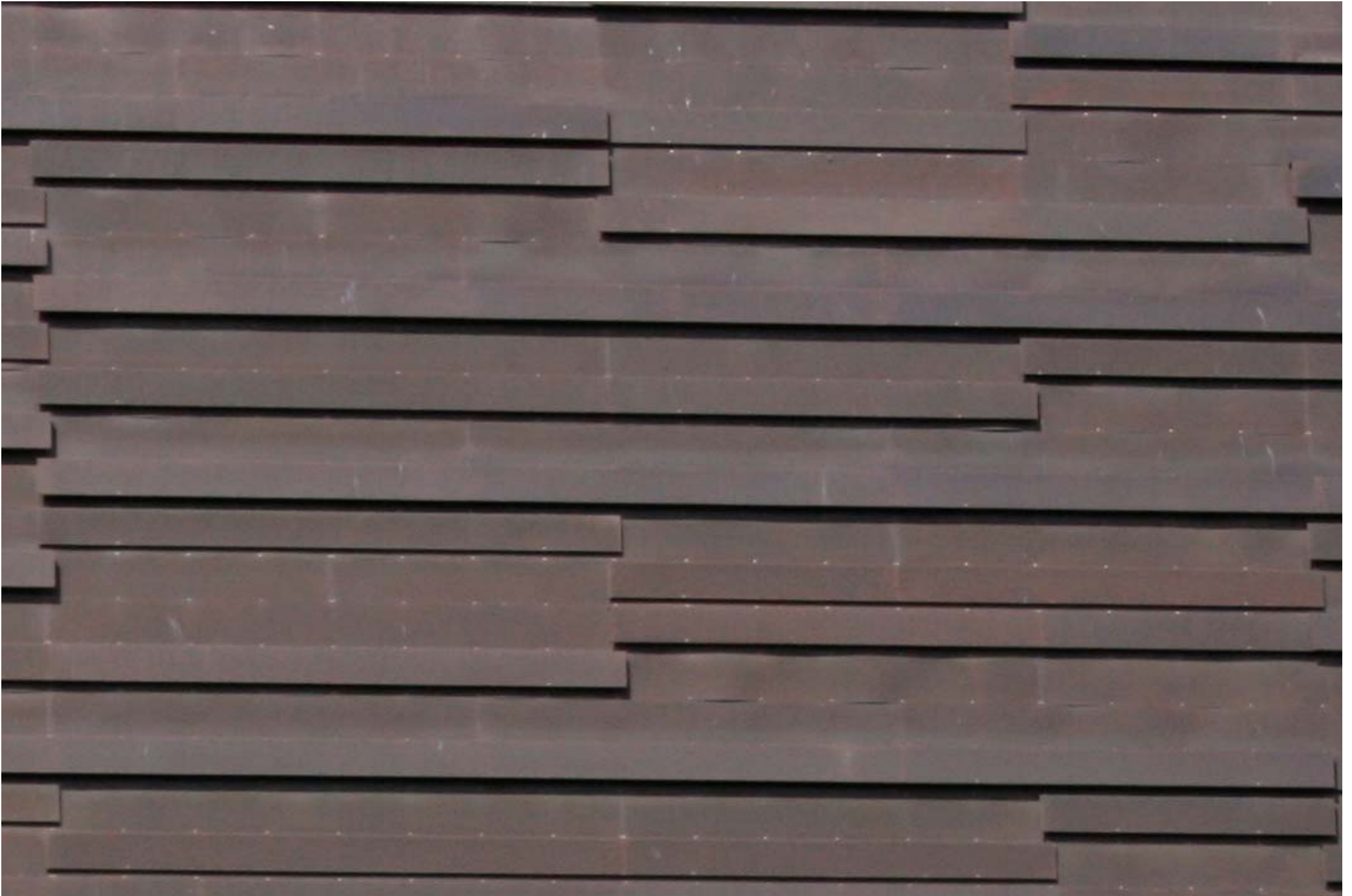
CONSTRUCTION & MATERIALS – Cooper clad fly tower
