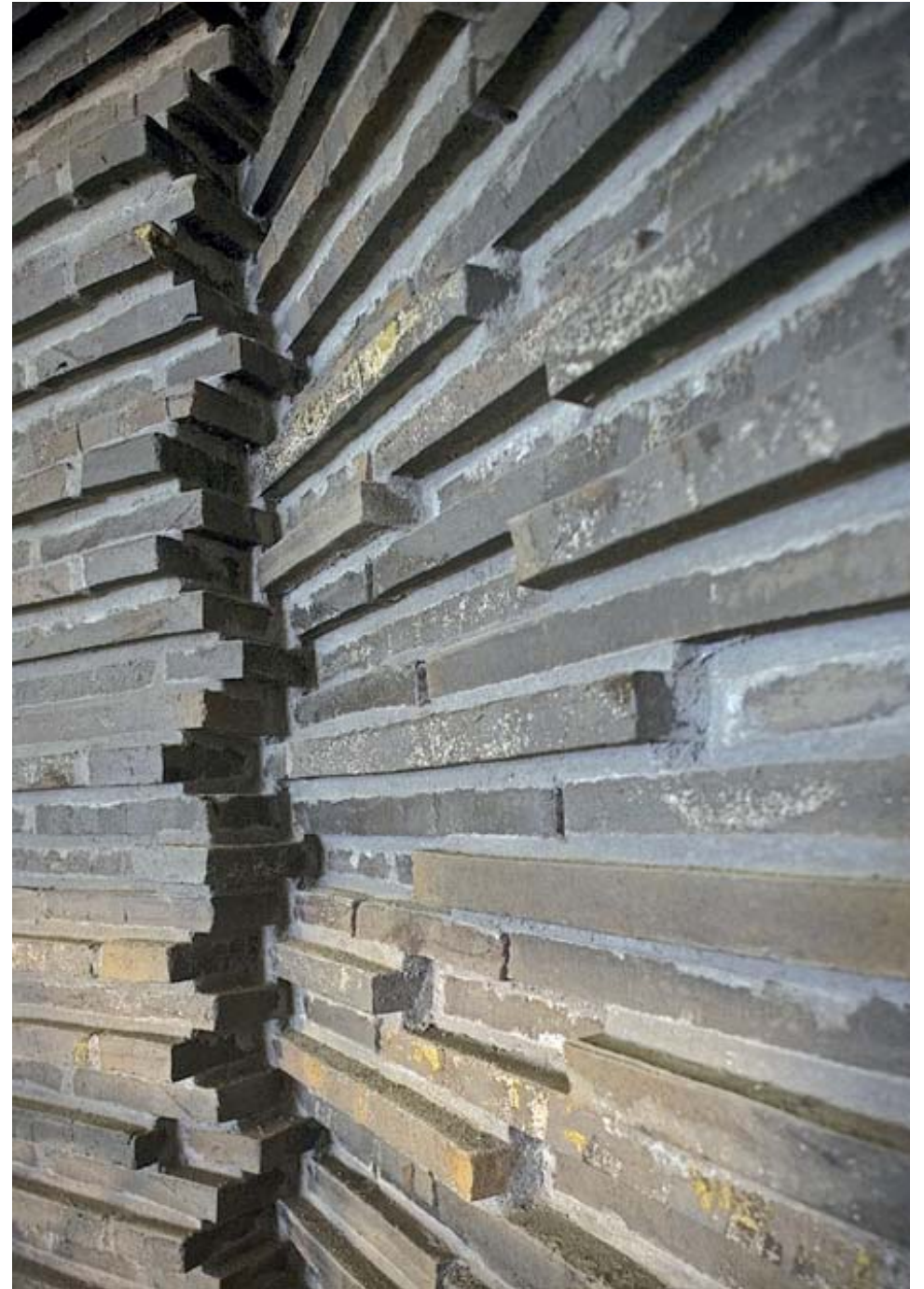
MATERIALS – Brick Auditoriums (External) – Handmade burnt english fireclay bricks
