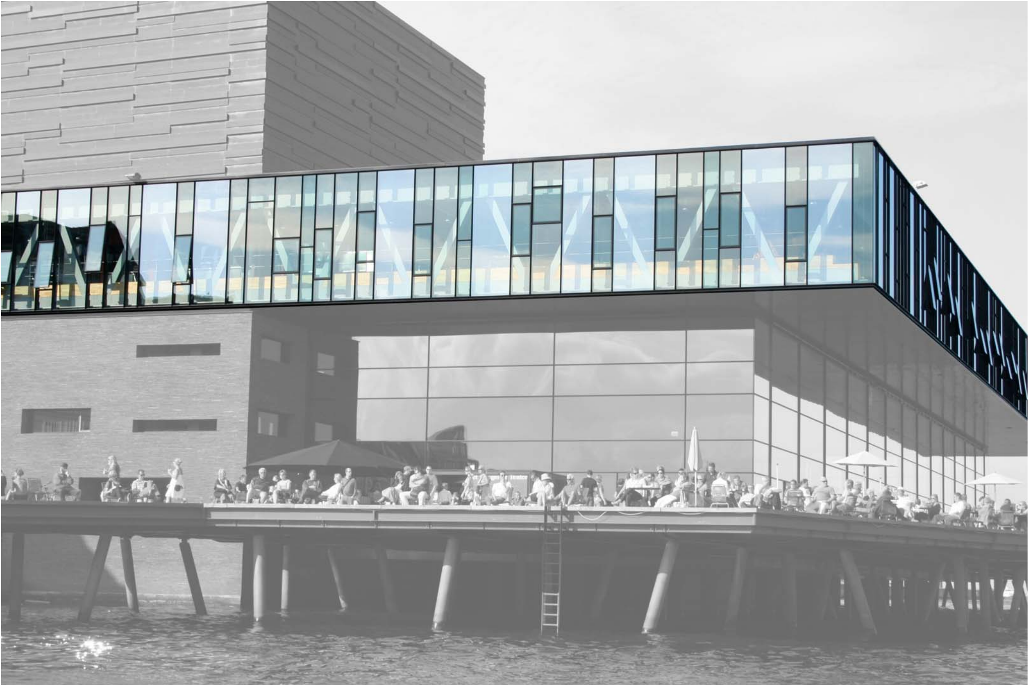
CONSTRUCTION & MATERIALS – Cantilevered all-glazed floor – working on display
