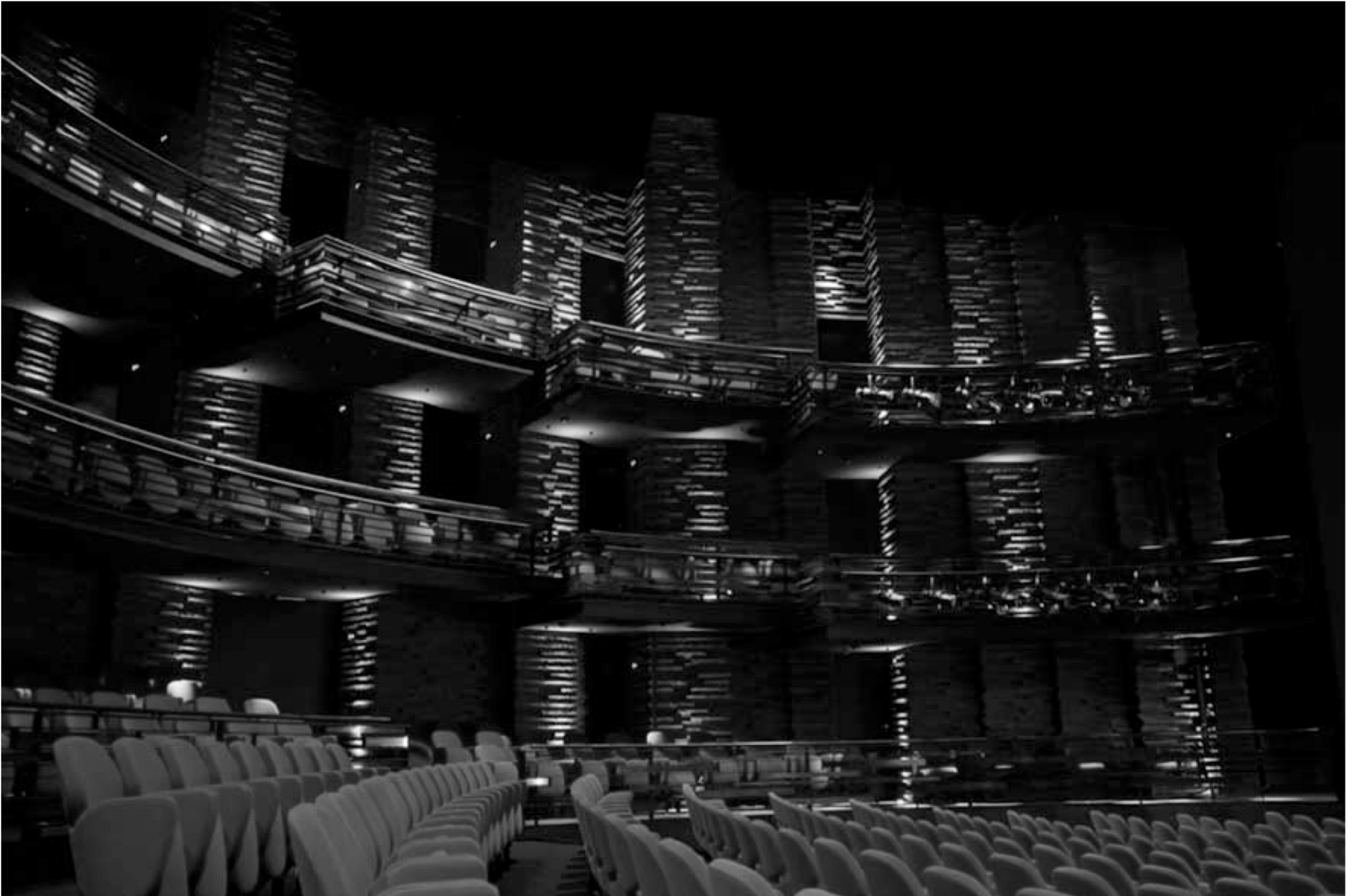
MATERIALS – Brick Auditoriums (Internal) – cliff-like, raw-energy and acoustics
