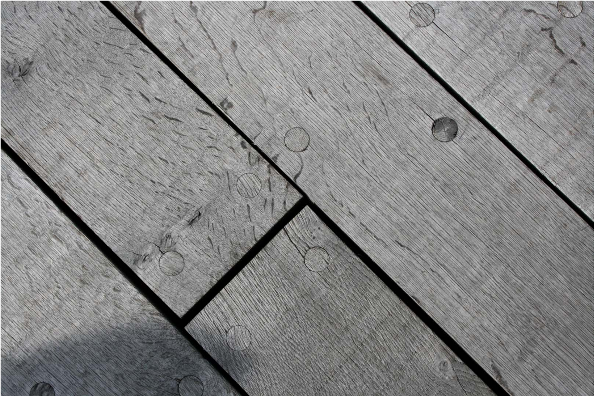
CONSTRUCTION & MATERIALS – Oak Promenade
