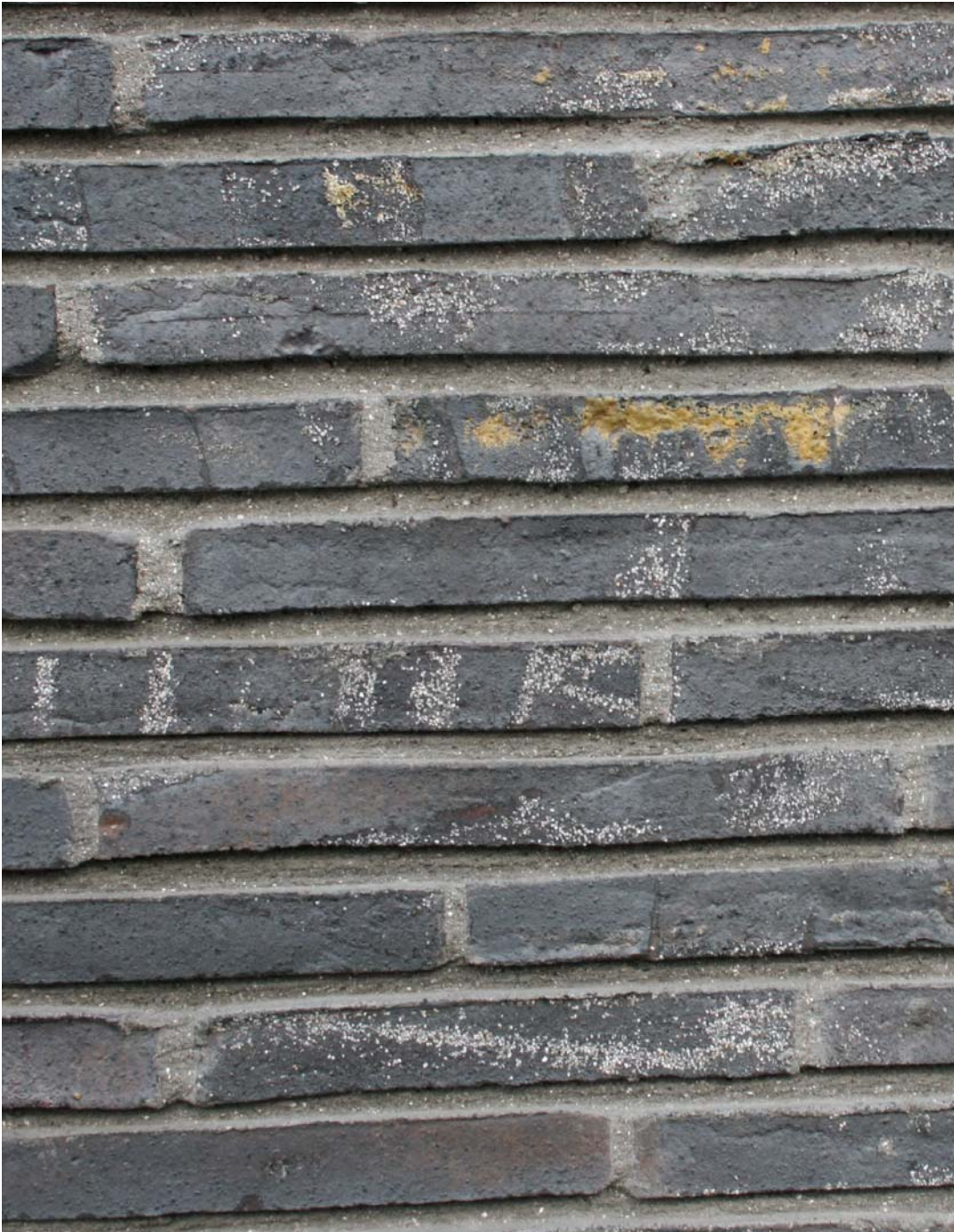
MATERIALS – Brick Auditoriums (External) – Handmade burnt english fireclay bricks
